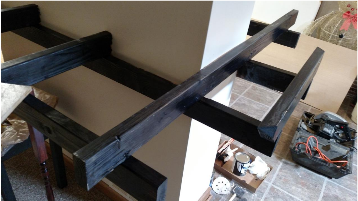
Ron's 2 x 4 construction is anchored to the duct chase structure
