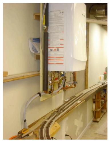
Editor Earl Paine's solution to an intruding hot water tank was to tear it out and replace it with a tankless unit. This created room for the trains to pass beneath the new unit and gain access to another basement area for a railroad extension.
