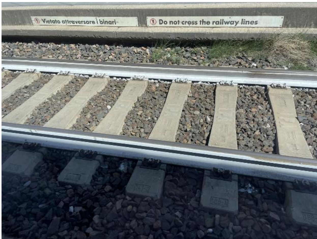
White painted rails on mainline welded trackage
