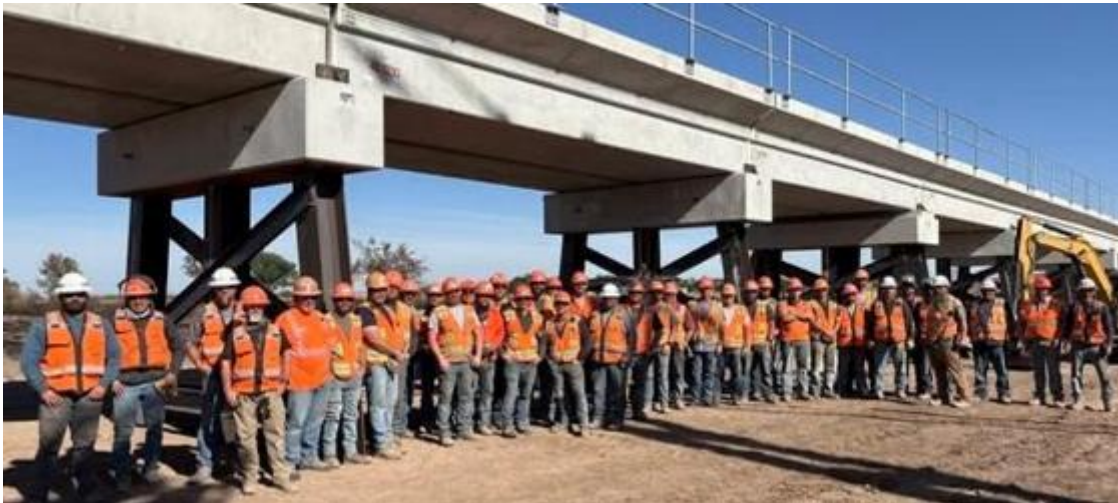
The new bridge is up and we have seen a picture of the first train going across it today!! Great, and fast work, to EVERYONE involved including the truck drivers and 3rd party contractors!! (Photo by BNST)
